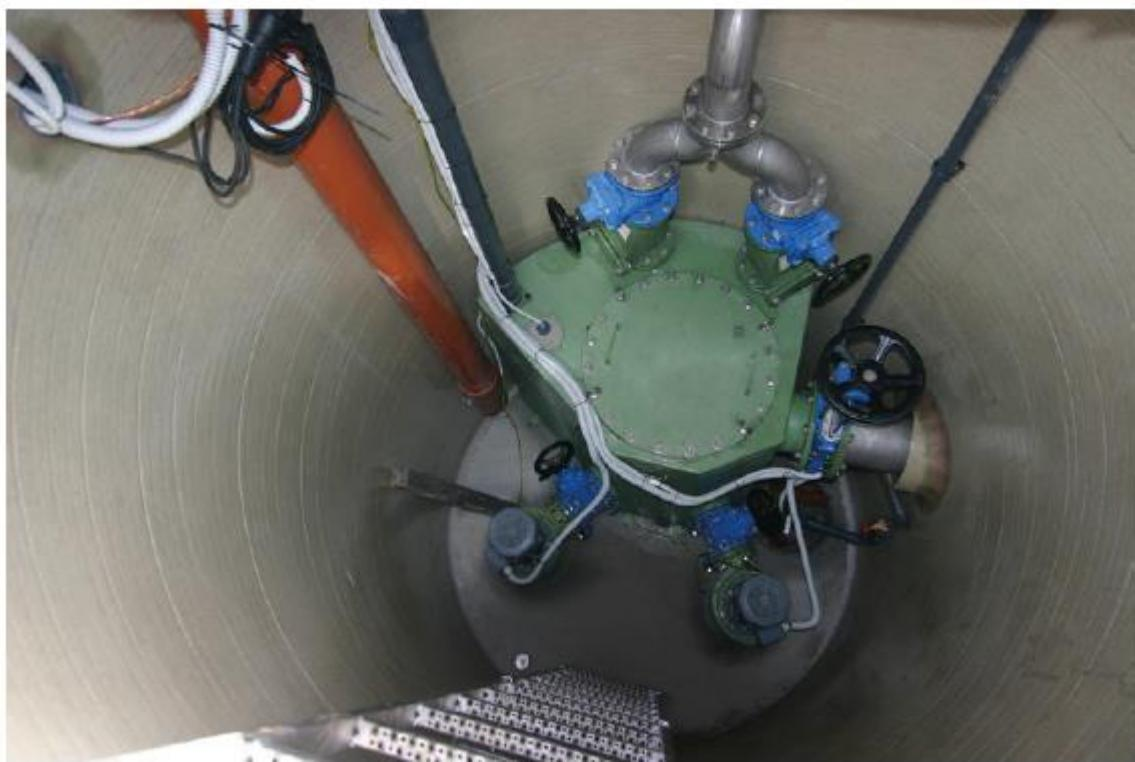
A mere 200m from the sea in Croatia this super Strate sewage installation handles all the sewage and also copes with the high salinity in the area by virtue of highly resistant anti-corrosion treatment. There, that's the technical bit.
