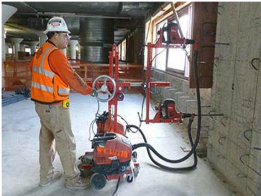
Contractors adopt innovative concrete drill jig to reduce silica exposures during concrete drilling operations. [Read more.](#)
