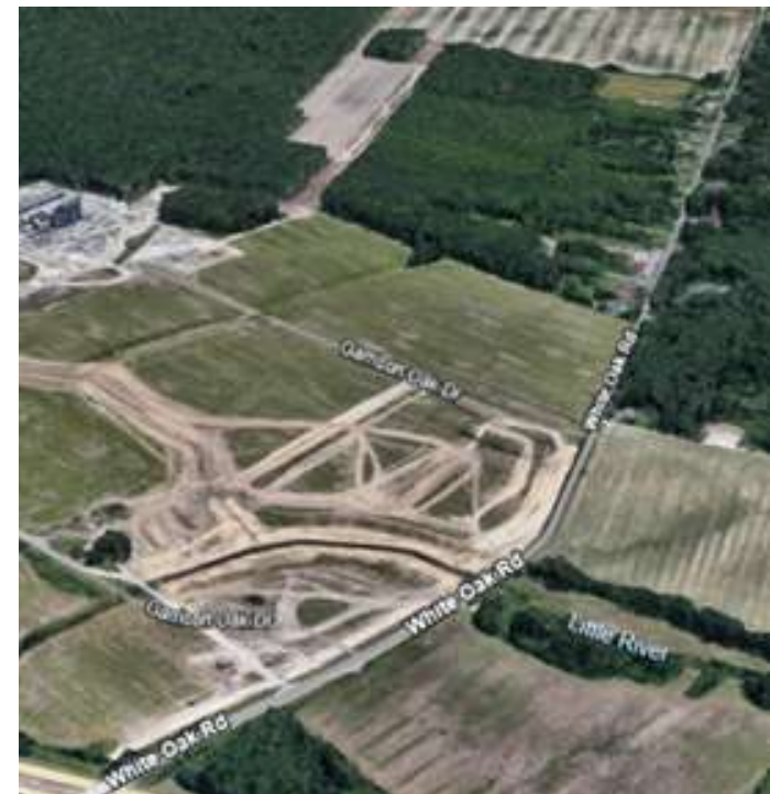
Aerial View of Garrison Oak Park
