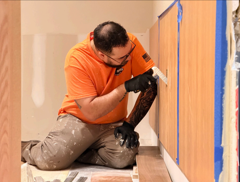
One of the many painters, Juan David, putting the finishing touches on the Commons’ new meeting room, DAN KING / THE GENERAL
