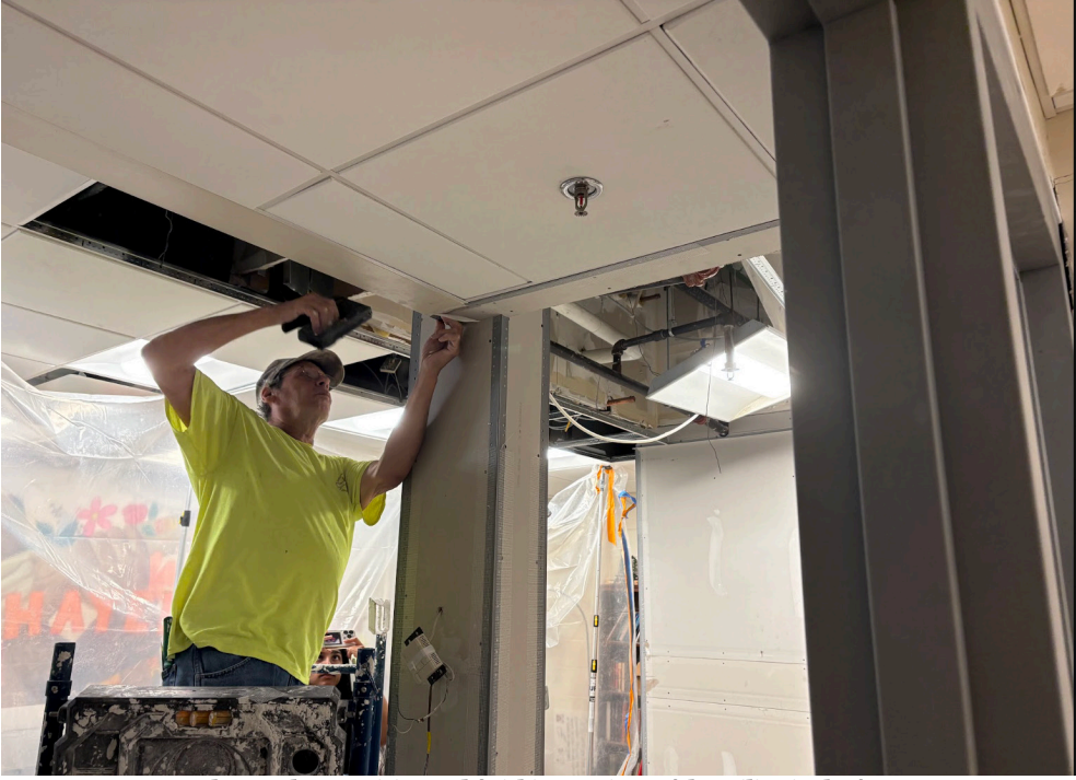
Another worker repairing and finishing sections of the ceiling in the former DEIB Lounge, AASHRITA JOGA, / THE GENERAL
