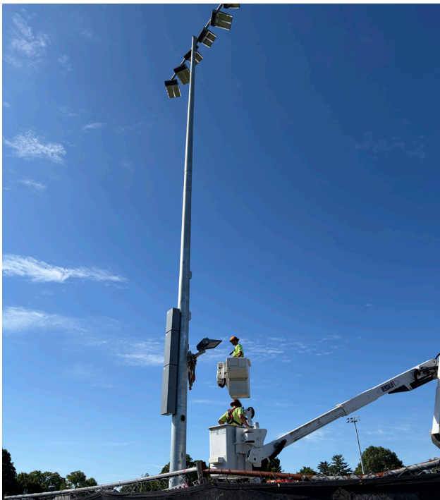
Workers construct the custom lights for the new football field in August, ANA SULLIVAN / THE GENERAL
