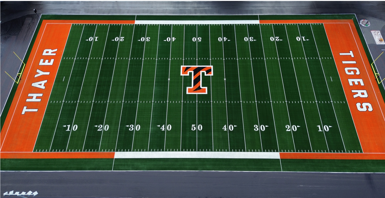
Thayer’s new multisport complex features a brand new turf field, a new track, new stands and press box, and an eventual “Tiger Tunnel”, DAN KING / THE GENERAL
