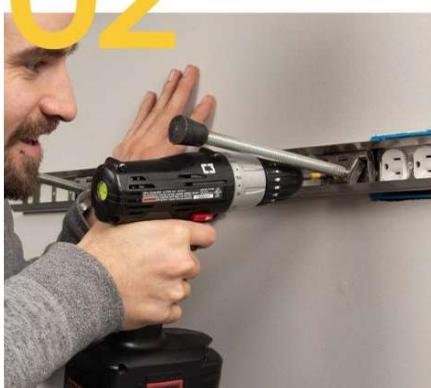
Find the wall stud with the studfinder and mark the wall in an inconspicuous place. Slide in the two brackets, and fasten them directly into the wall stud.
