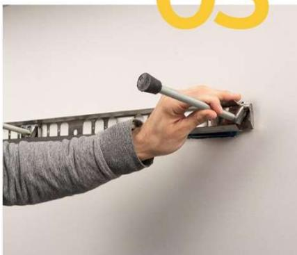
Level the brackets by rotating the rods. Place the level on the tip of the bracket rod and on the rail, and rotate the rod as necessary.
