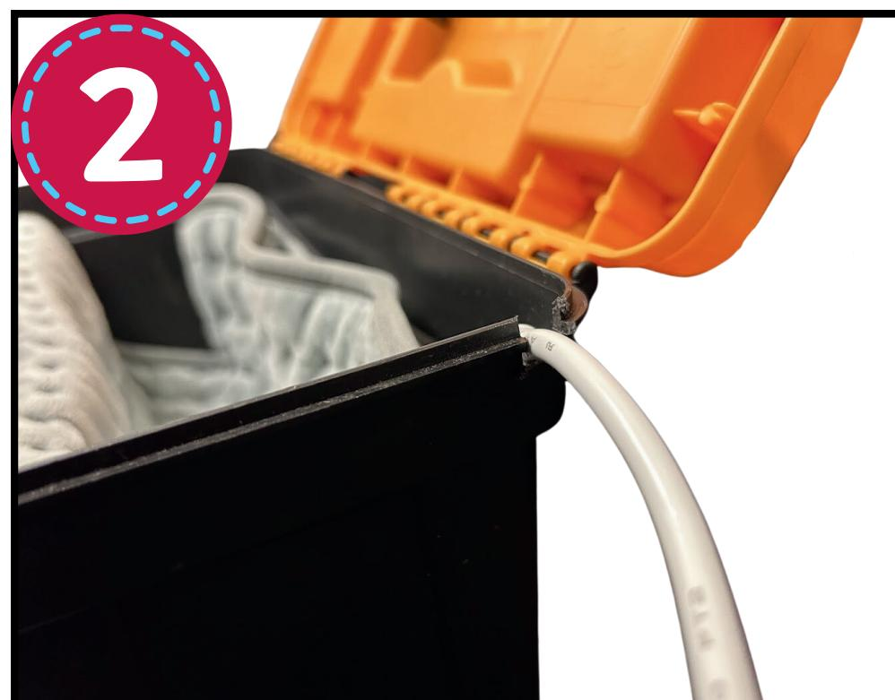
Cut a notch into the toolbox
