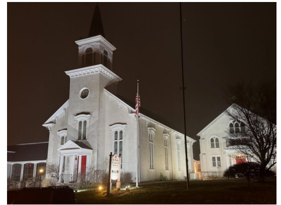
Church Lighting, March 7, 2026
