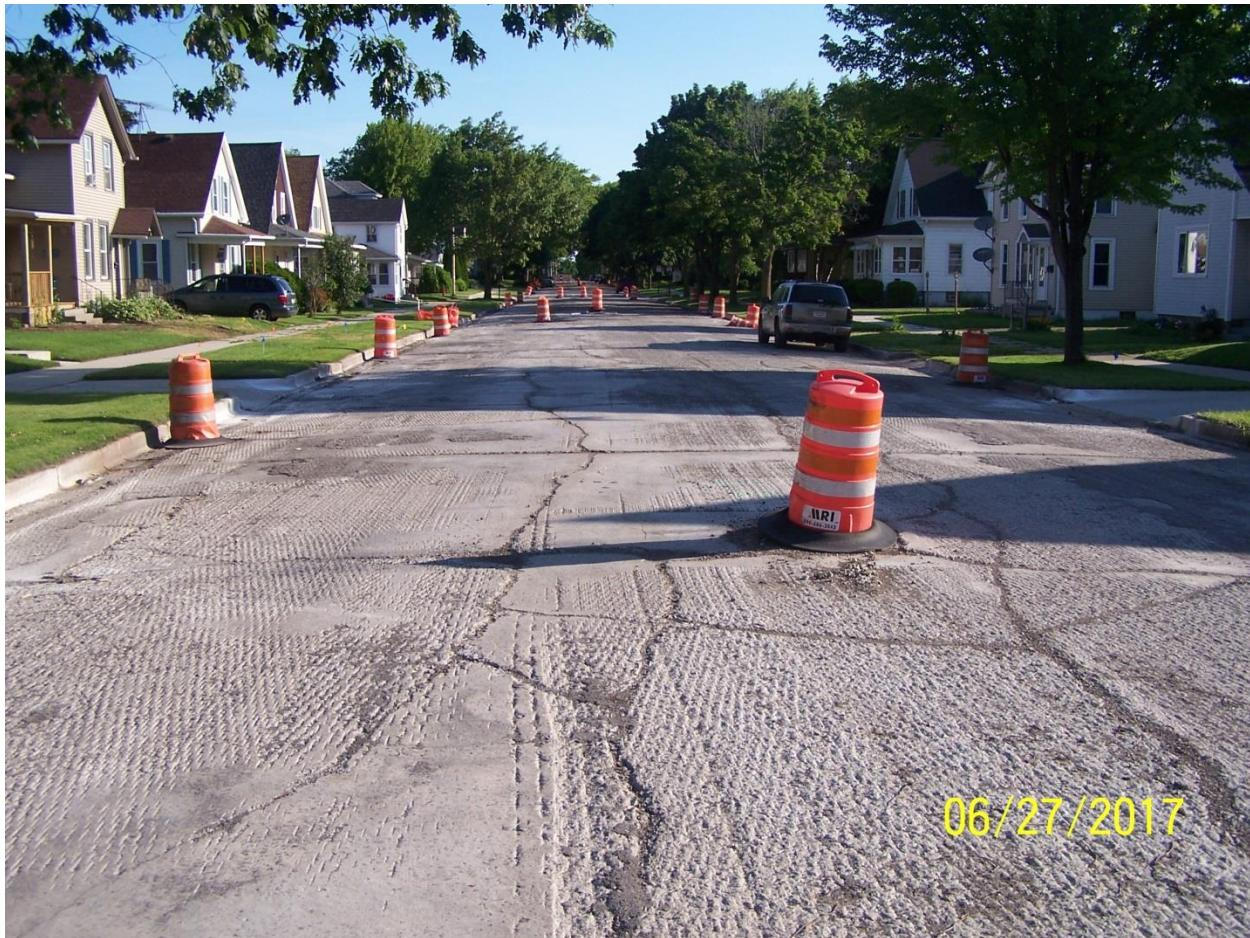
All of the utility work has been completed on North 10<sup>th</sup> Street between Superior Avenue and Geele Avenue. Curb and gutter removal and replacement will start the week of July 3<sup>rd</sup> and will be completed the week of July 10<sup>th</sup>. All sidewalk and curb ramps at the intersections will also be completed in early July. By the end of July, all asphalt paving should be completed by City of Sheboygan Public Works.
