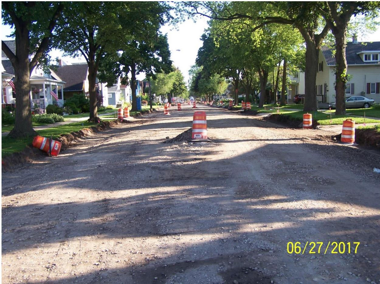
All of the utility work has been completed on North 12th Street between Superior Avenue and Geele Avenue. Curb and gutter removal and replacement will start the week of July 3<sup>rd</sup> and will be completed the week of July 10<sup>th</sup>. All sidewalk and curb ramps at the intersections will also be completed in early to mid-July. By the end of July, all asphalt paving should be completed by City of Sheboygan Public Works.
