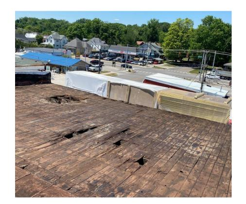
Holy moly! No wonder the roof was leaking like a sieve. The decking was so rotten that a large area had to be demolished and completely rebuilt.
