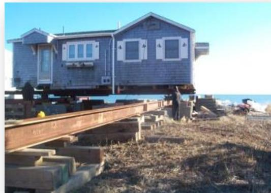
**Case Study 2:** Release of 150 gallons of heating oil to earthen crawl space beneath home on Cape Cod. The resulting cleanup costs for contaminated soil removal, groundwater treatment, and moving the home to excavate impacted soil cost more than \$200,000. The homeowner had insurance that covered all but \$10,000 of the work.
