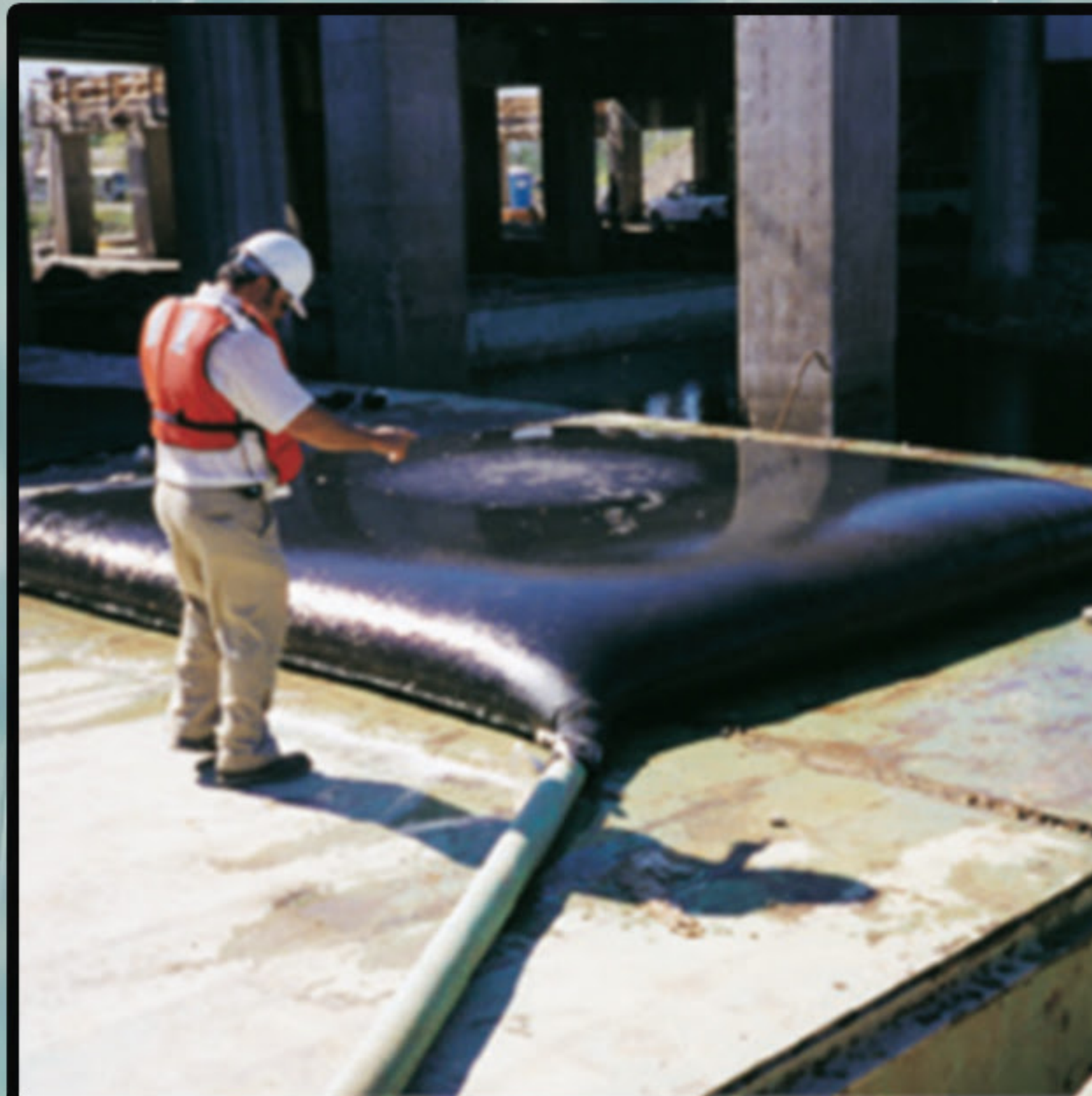
SILT/SEDIMENT SACKS
