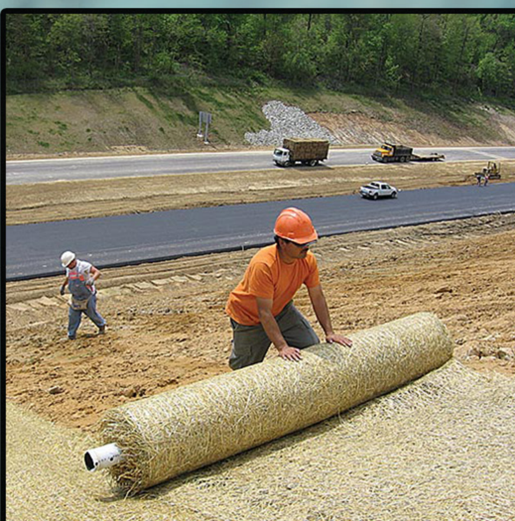
STRAW EROSION CONTROL BLANKETS IN 7.5' X 120' ROLLS
