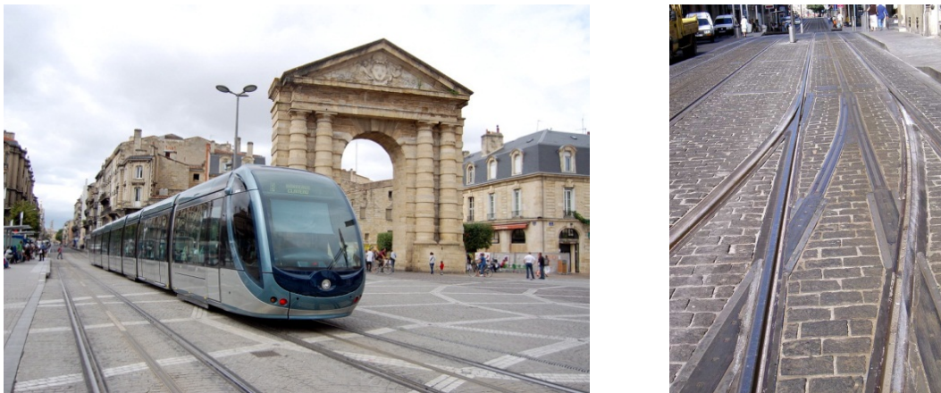
FIGURE 4-5 Ground Level Power System
