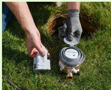
Advanced Metering Infrastructure (AMI) is capable of collecting and reporting water use data in real-time, providing timely information about water usage to both the city and water customers.
