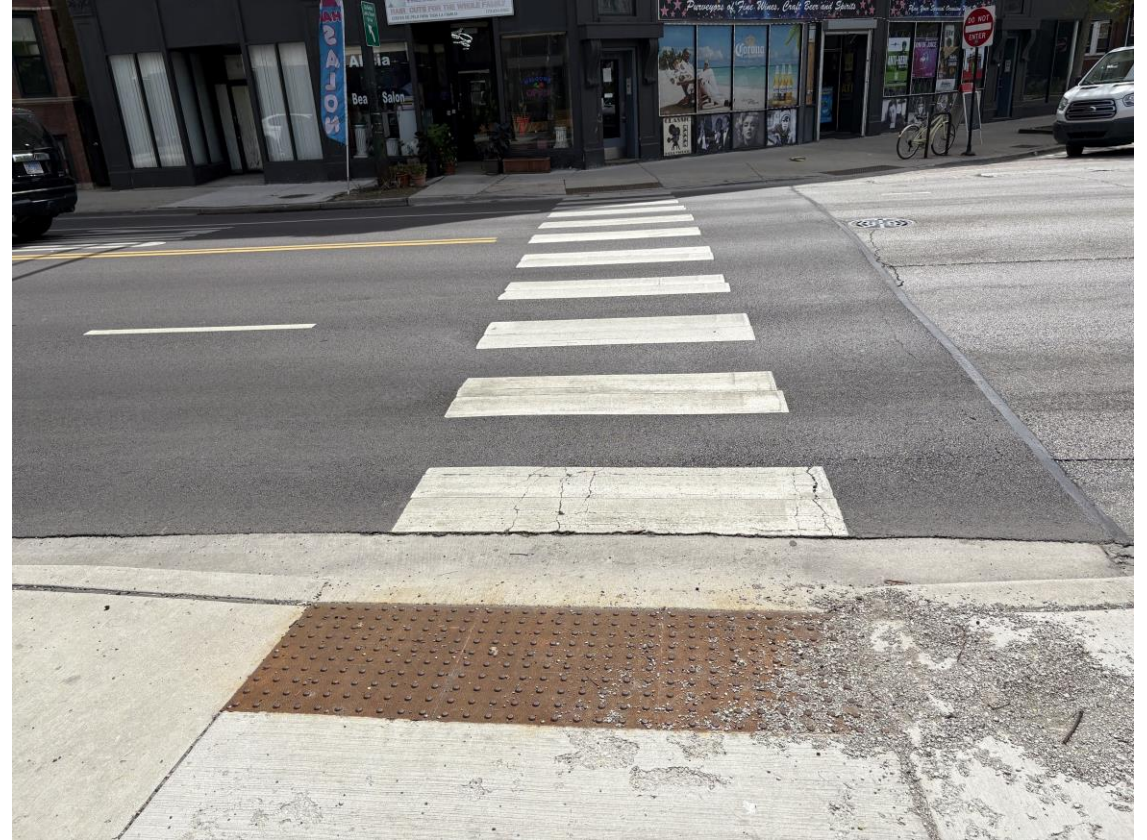
SOUTH CROSSWALK ON RIDGE LOOKING WEST
