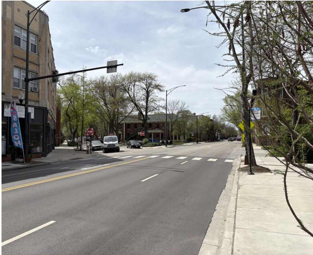
NORTHBOUND LANES ON RIDGE LOOKING NORTHWEST
