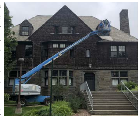
Restoration of 3rd floor dormer windows
