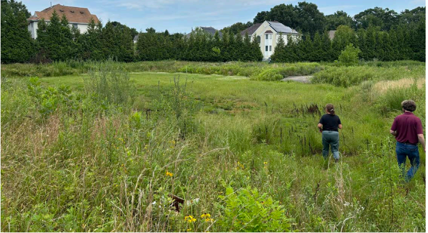
Tuscan Terrace Stormwater Basin retrofitted with native grasses and perennials.
