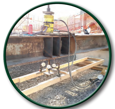
Pile load testing
