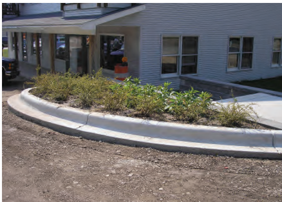
Top: A low-impact storm sewer installed in the City of Grayling significantly reduced the discharge of untreated stormwater into the AuSable River.
