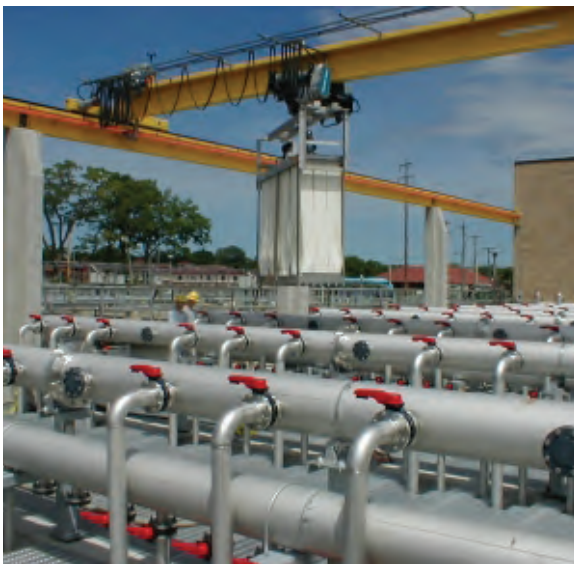
Top: The Village of Kalkaska's new 600,000 GPD Wastewater Treatment Plant is capable of expansion for future growth.
