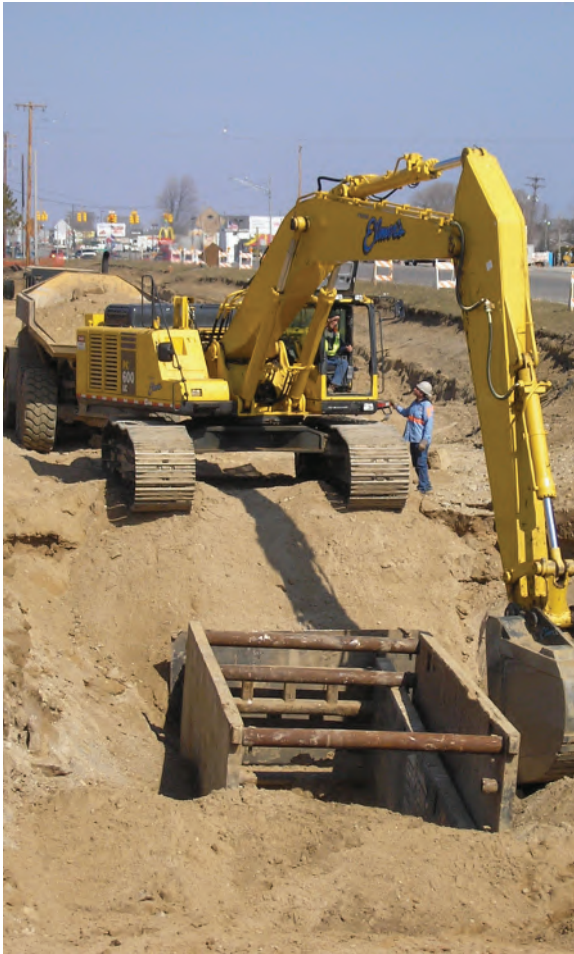
Gosling Czubak designed ten miles of gravity sewer and five miles of force main to serve the growing Blair Township in Grand Traverse County.
