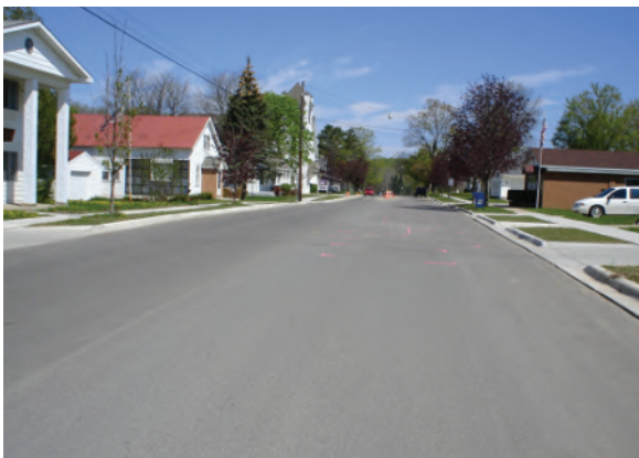
Top: Gosling CZubak completed construction engineering of a nearly 4-mile stretch of Spencer Road through Kalkaska County.
