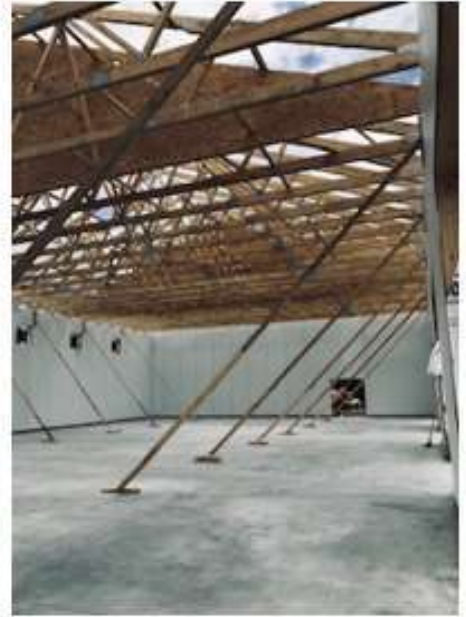
Temporary bracing
