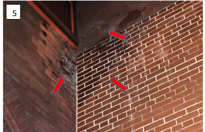
Efflorescence has developed on peak area of arch, under the arch and on the east side of arch, tuckpointing and masonry cleaning recommended (pic 6)
