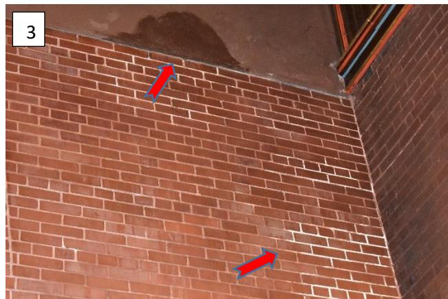
Northside (to the left of arch center) visible wet spots on plaster section of masonry, swollen, separating from the wall and crumbling plaster. Wet spots on brickwork, deteriorated brick, efflorescence on brick joints, Brick replacement, tuckpointing, masonry cleaning, plaster section replacement recommended (pic 4,5)
