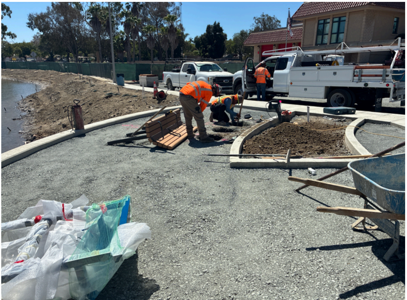
Photo: Installing footers for site furnishing.
