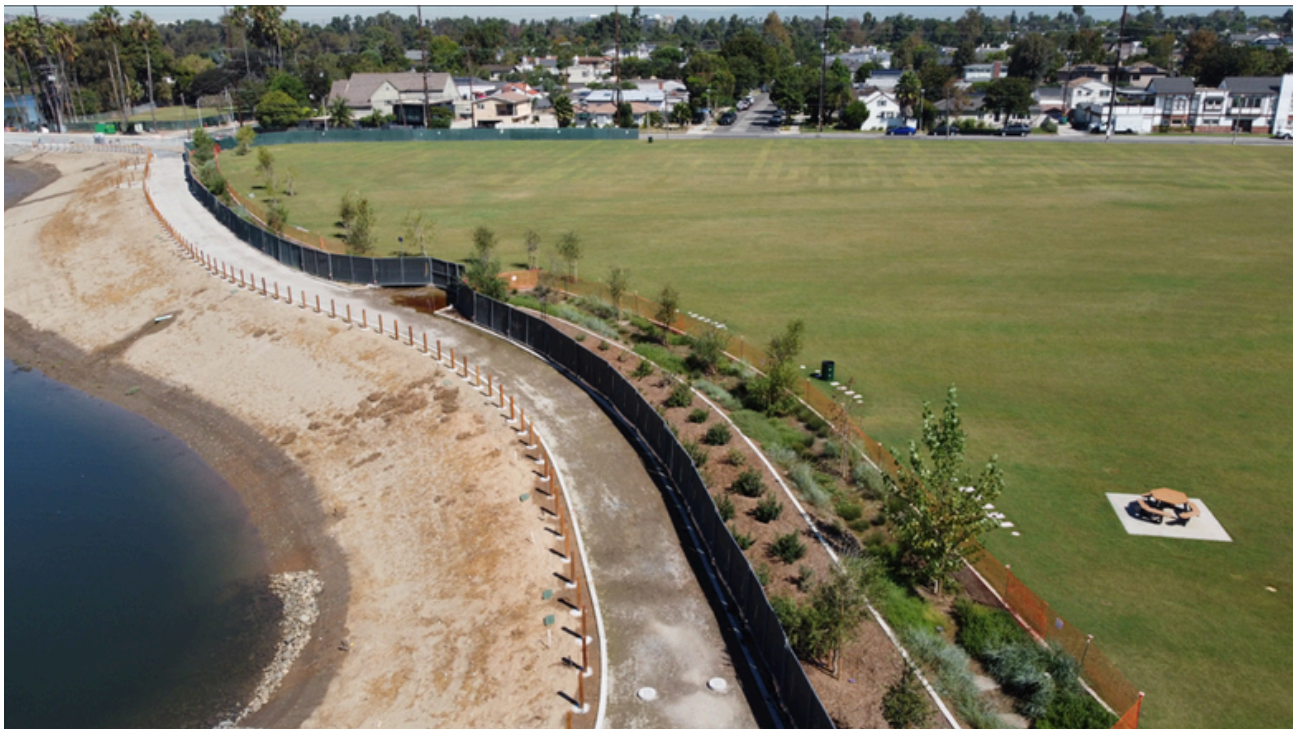
Photo: Base maPhoto: Preparing for final decomposed granite (DG) path installation.terial.
