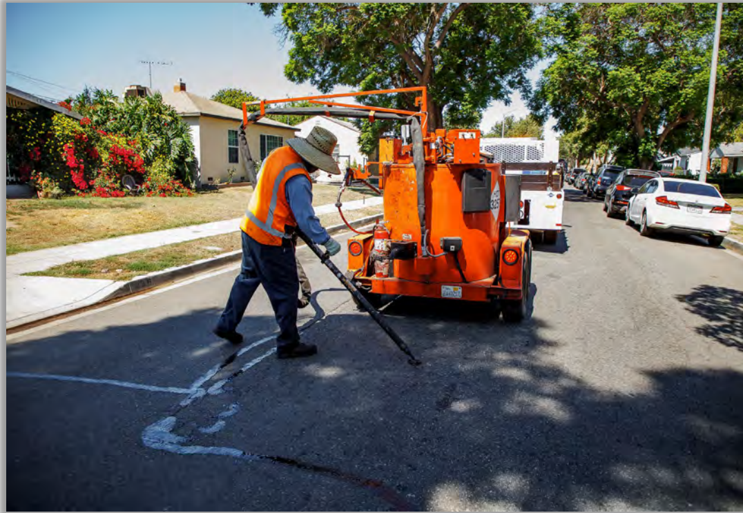
Crack Seal
