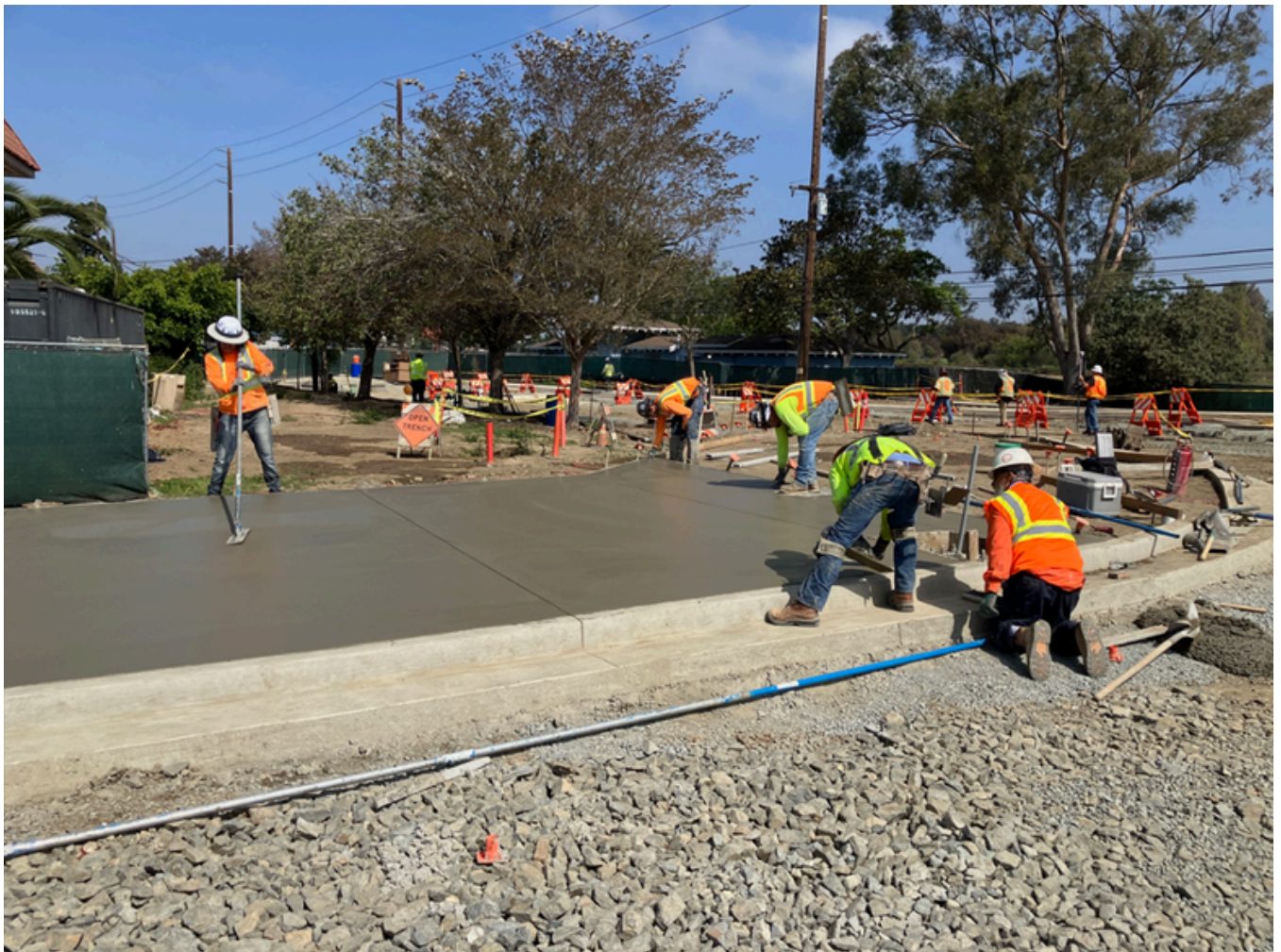
Photo: Sidewalk installed at Colorado at Eliot and curing in progress.
