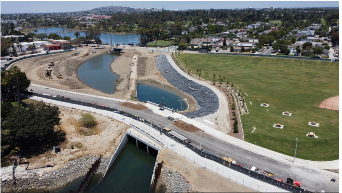
Photo: June 23, 2026 aerial of Marina Vista Park and Open Channel construction.
