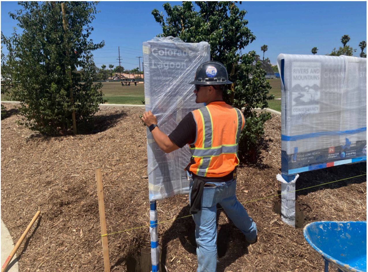
Photo: Park and trail signs being installed.
