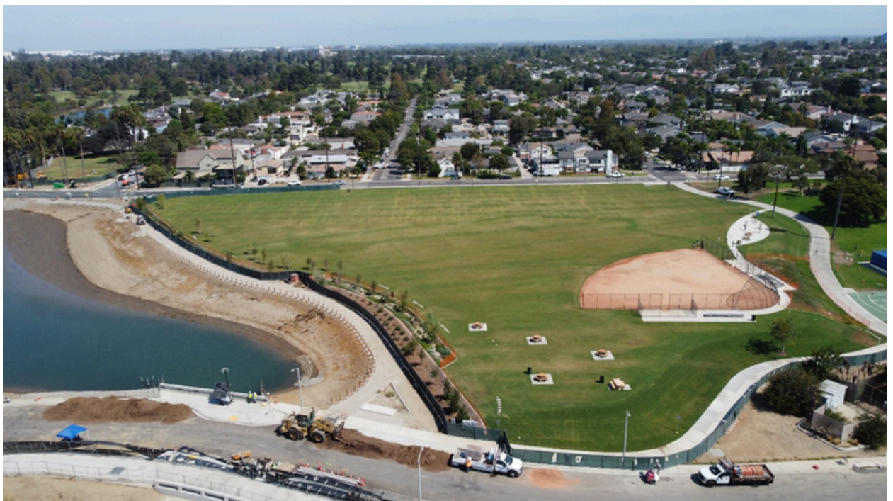
Photo: Aerial image from August 25, 2026
