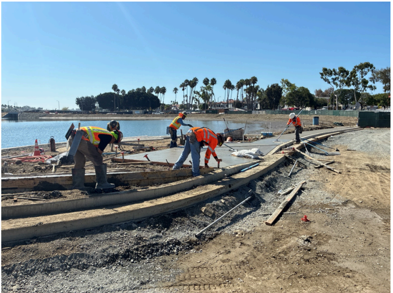
Photo: Sidewalks and curb ramps installation
