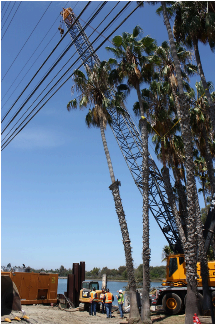
Photo: Crane was relocated and staged at Alamitos Heights Park
