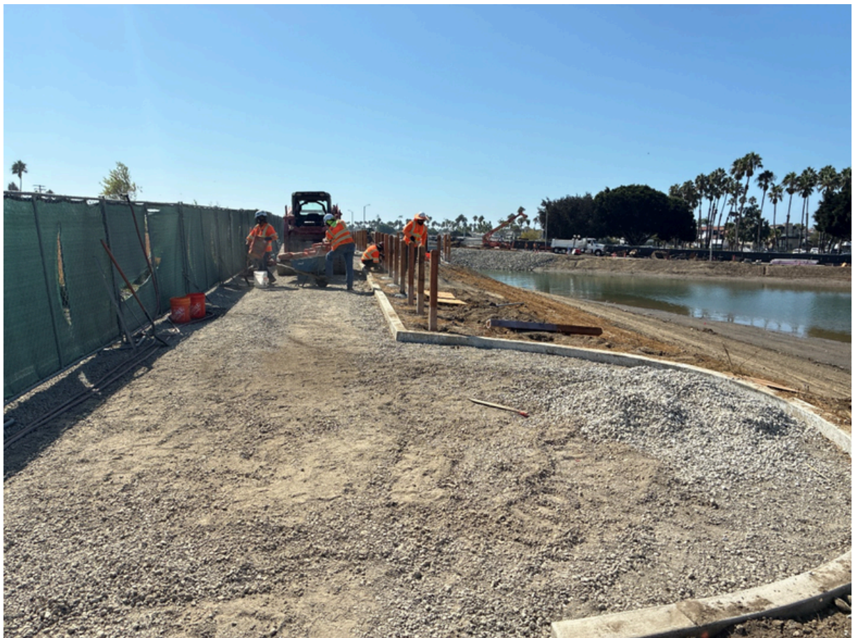
Photo: Fencing (log and wire) base of posts set into concrete
