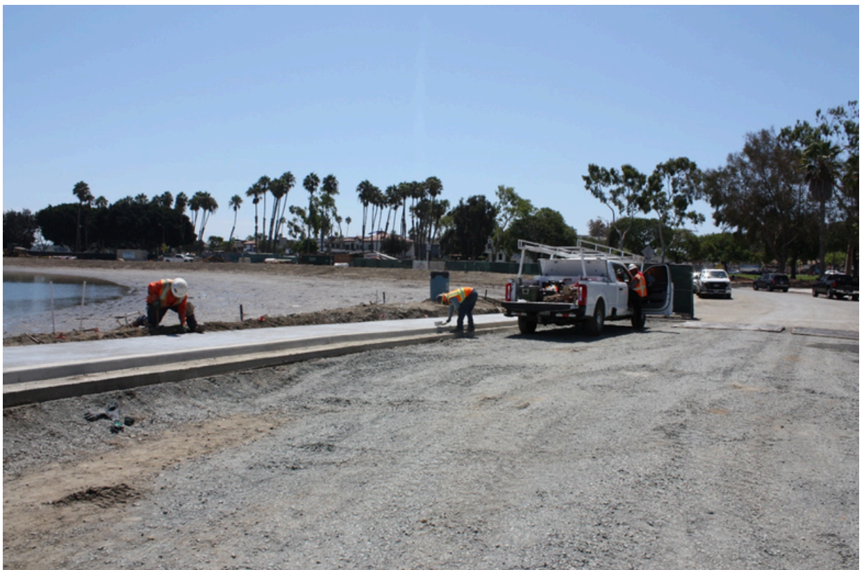
Photo: Finishing concrete work
