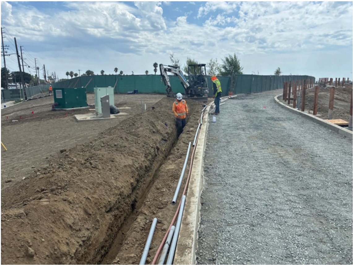
Photo: Irrigation line installation
