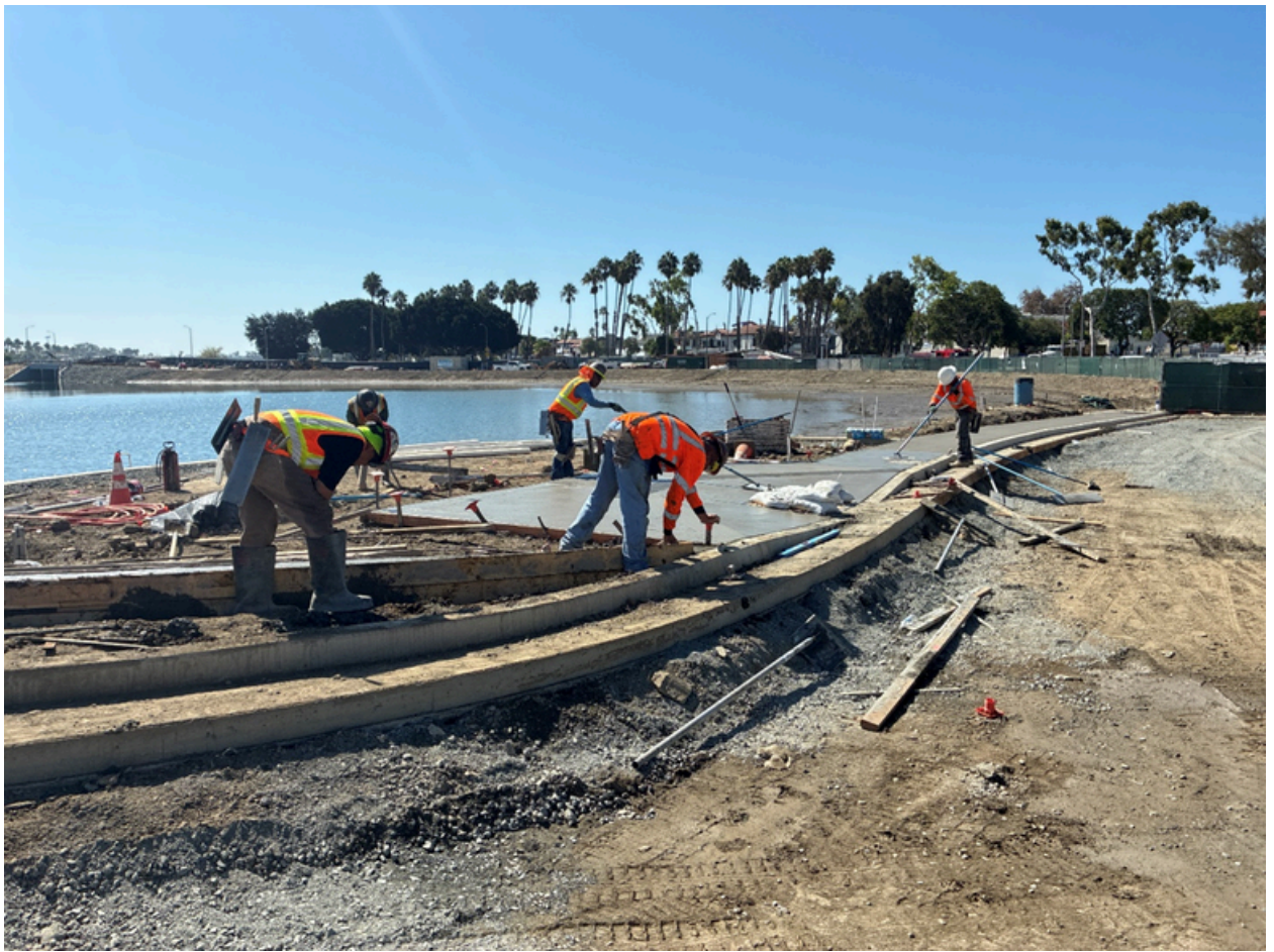
Photo: Sidewalks and curb ramps installation
