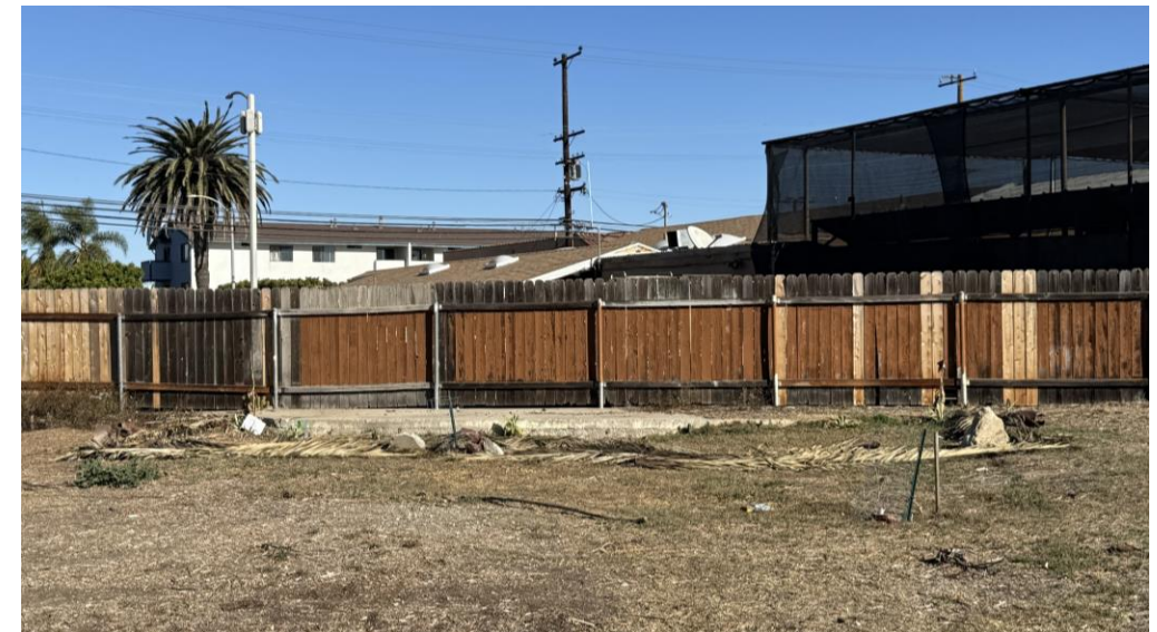
Fencing, concrete pad
