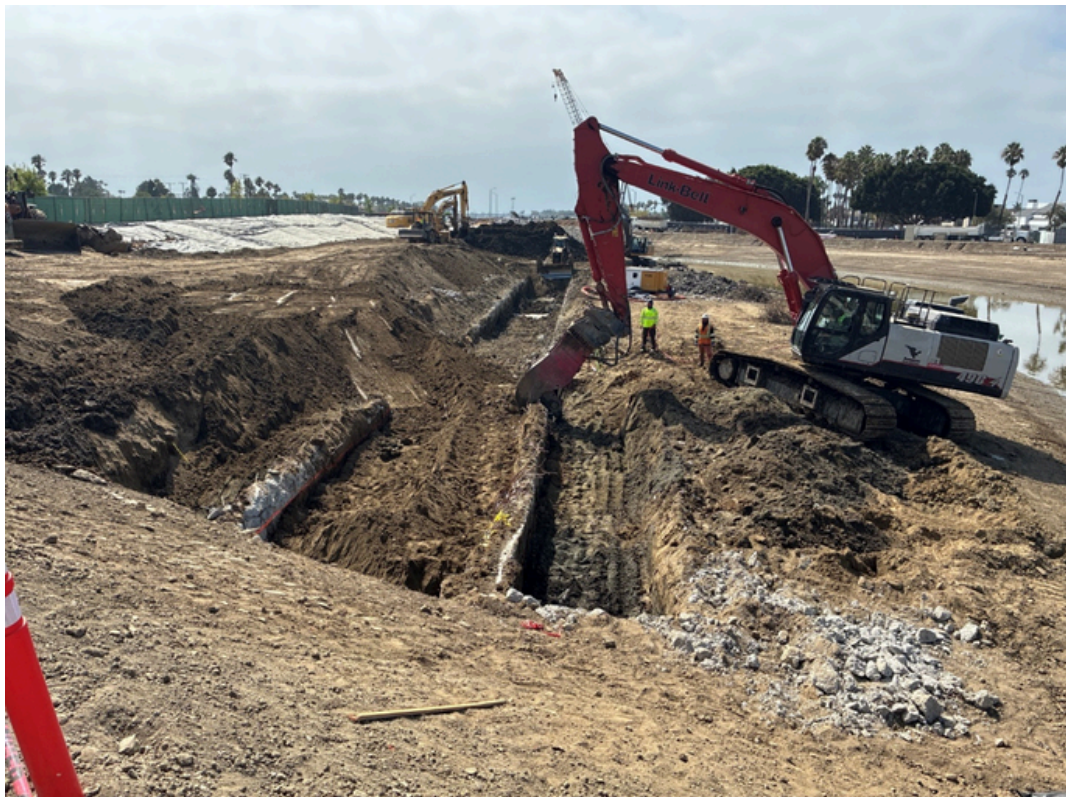
Photo: Culvert demolition in progress
