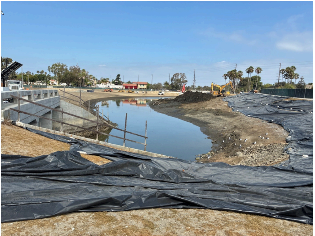
Photo: Recent photo of culvert mostly removed and concurrent grading
