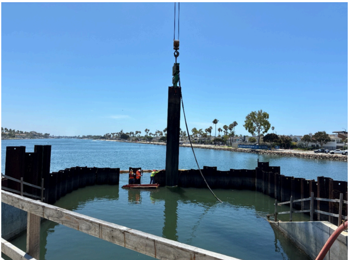
Photo: Added new sheet piles to restrict water flow to advance culvert demolition work
