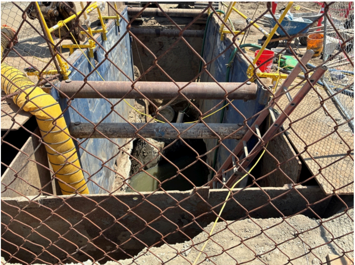
Photo: Shoring to support installation and connection of remaining storm drain lines
