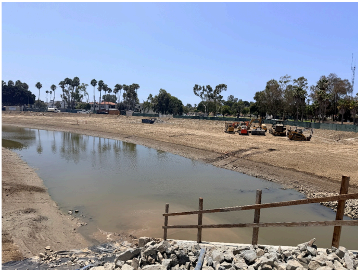
Photo: Grading of the west bank of the open channel
