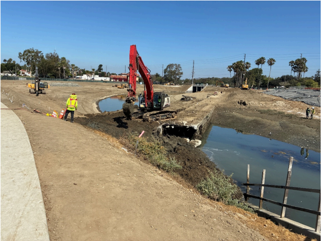
Photo: Culvert demolition initiating
