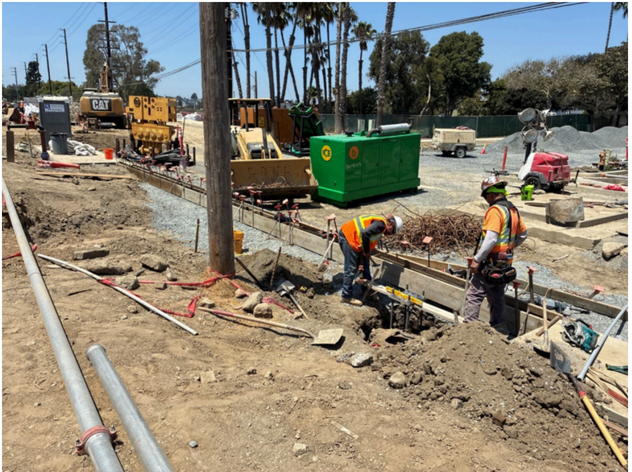
Photo: Crews installing forms in preparation for concrete placement for additional curb sections
