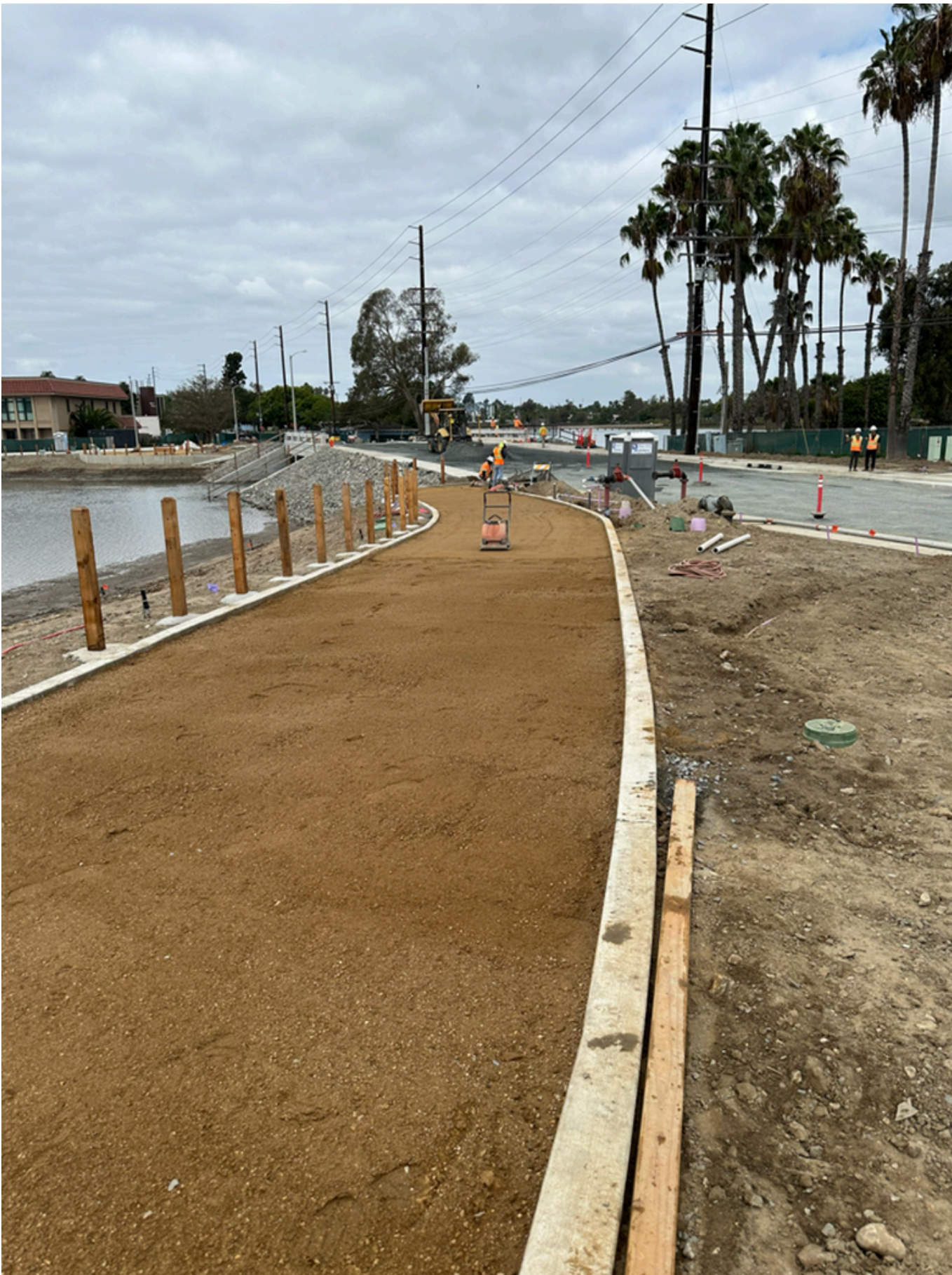
Photos: DG installation and compaction in progress.
