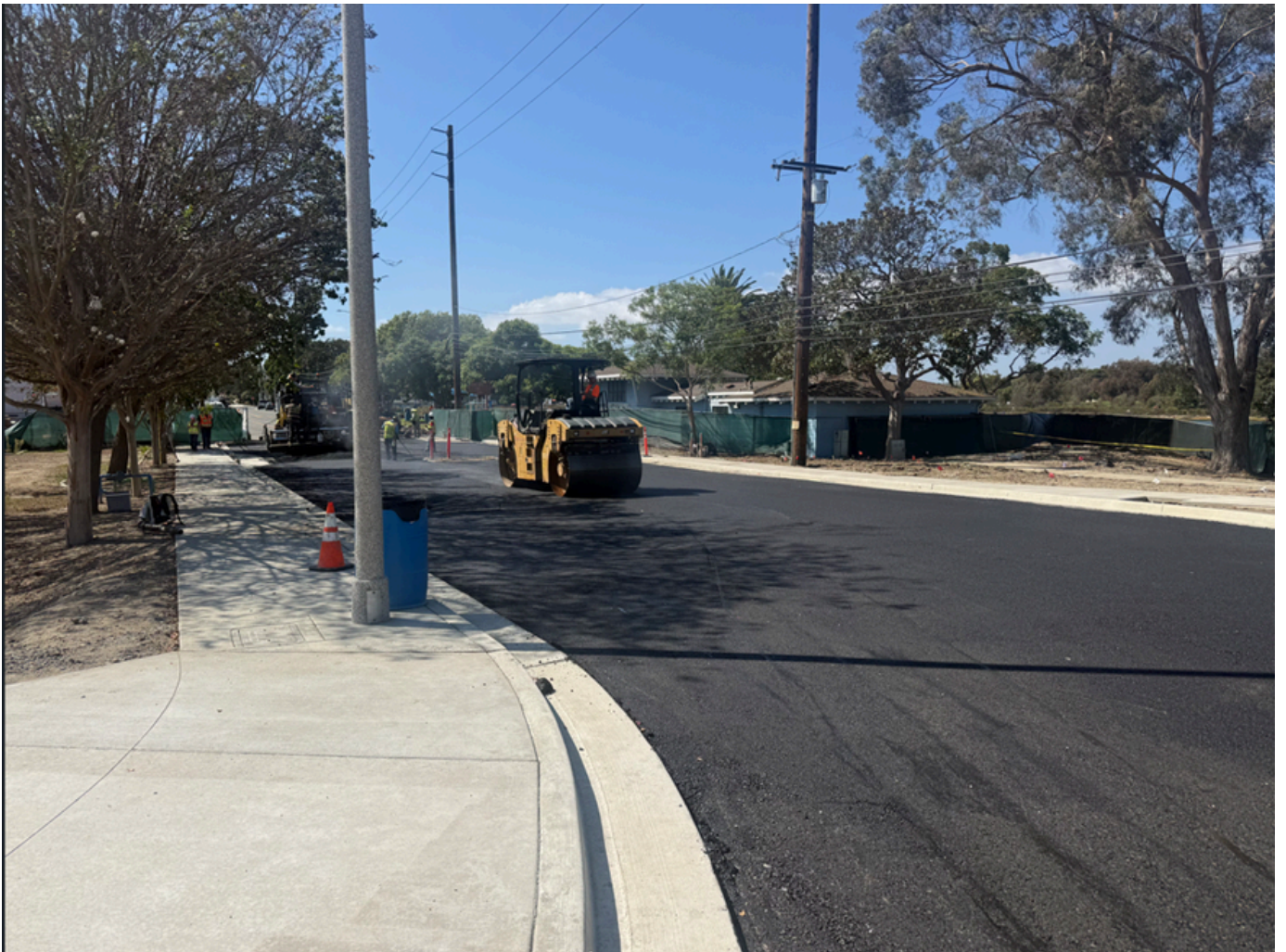
Photos: Asphalt paving installation.
