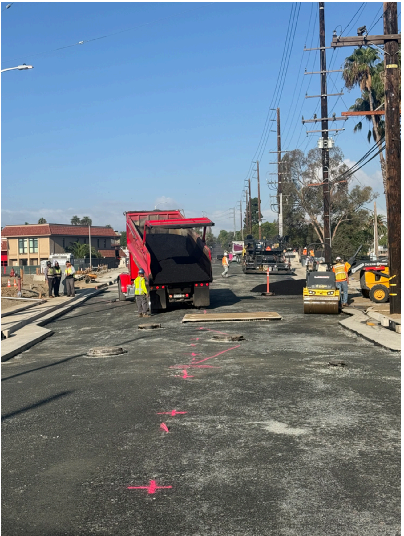
Photos: Asphalt paving installation.
