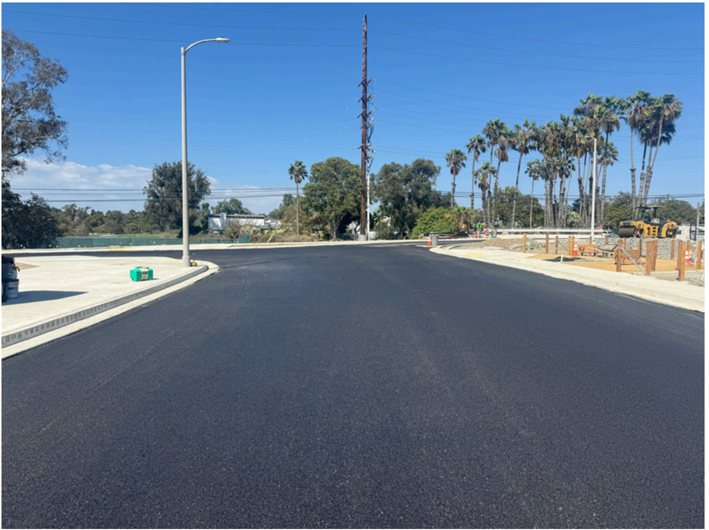
Photos: Pending final course of pavement.
