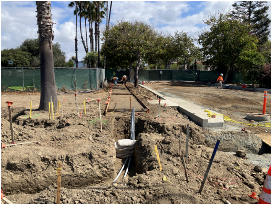
Photo above: Trenching and installation of conduits for street lights
