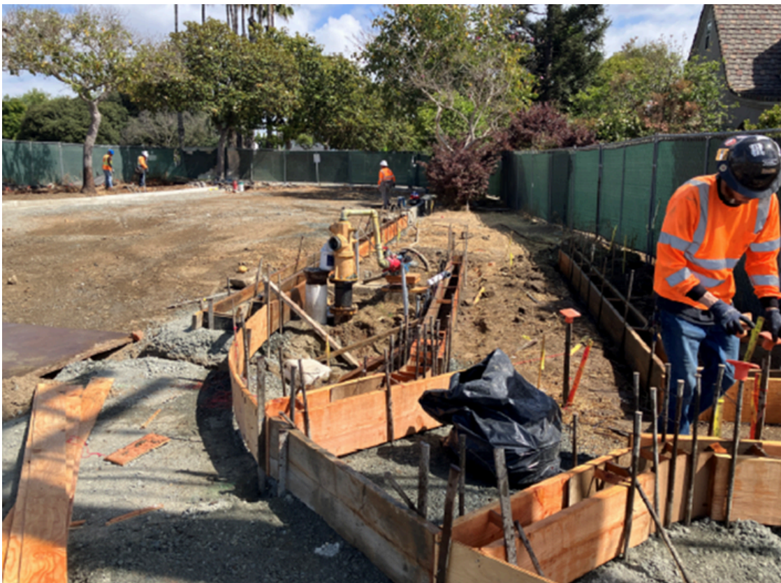
Photo above: Orlena curbs / gutters and rebuild on-going
