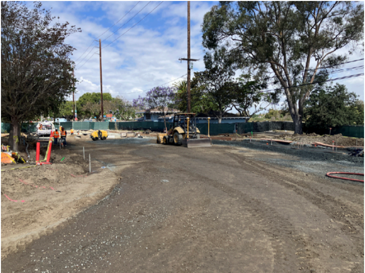
Photo above: limport and placement of base material for sidewalks, curbs and gutters at Colorado Street began.
