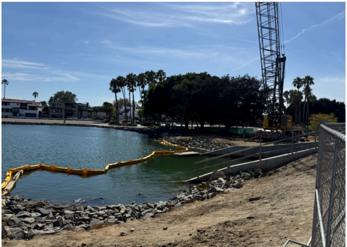
Photo: Removal of sheet piles completed at Eliot Street and rip rap installed
