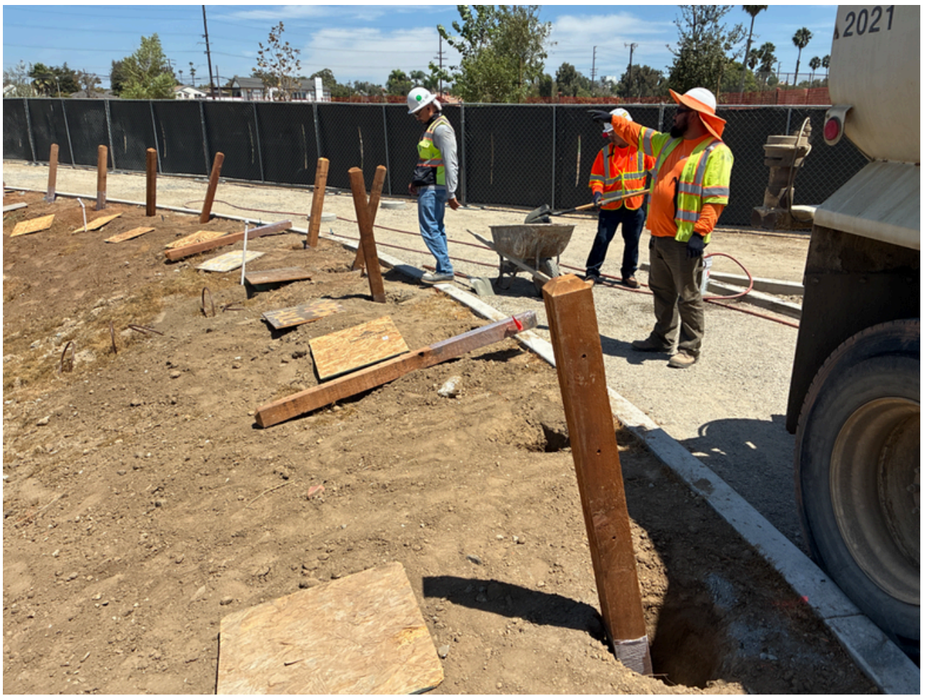
Photo: Log and wire fence system being installed
