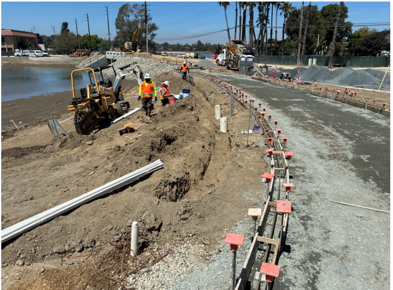
Photo: Crews continue with the installation of irrigation lines to support future planting
