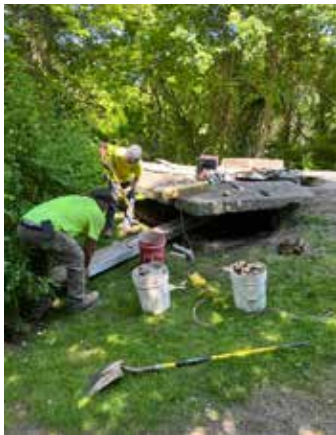
Employees of the Joseph Gnazzo Co. stabilizing the roof of a World War I observation post.
