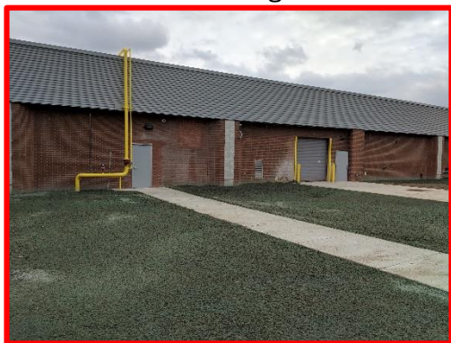
Picture 2: Exterior Progress at the North Entrance
