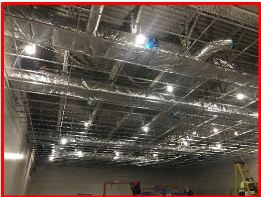
Picture 2: Ceiling Grid in the LGIA
