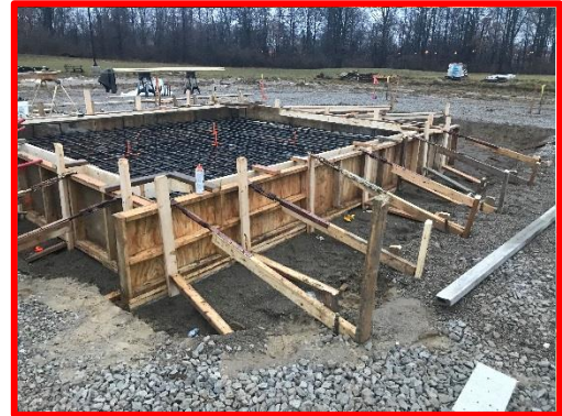
Picture 5: Reinforcing Steel for the Burn Building Foundation
