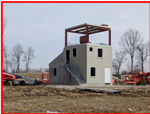
Picture 4: Exterior Finishes on the Burn Building
