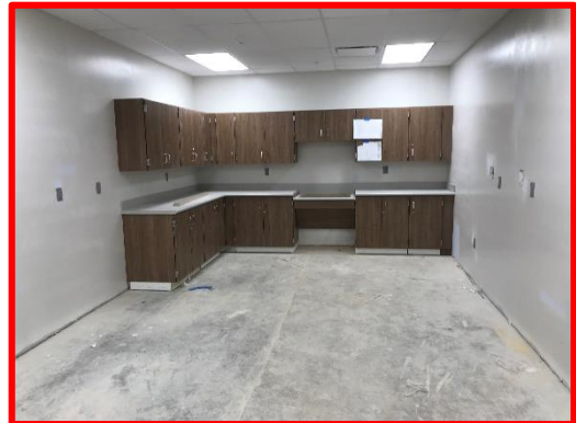
Picture 7: Casework in the East Prep Kitchen
