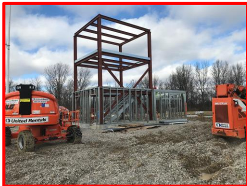
Picture 2: Burn Building Progress
