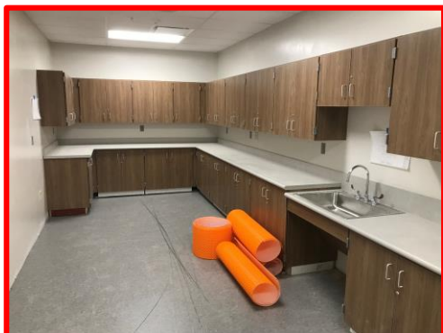
Picture 3: Casework and Vinyl Composition Tile in the East Admin Workroom
