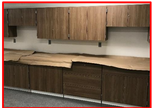
Picture 7: VCT and Casework in the General Science Classroom
