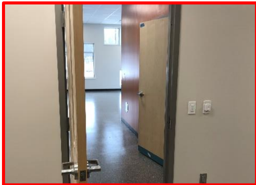
Picture 4: Doors Installed in the Early Childhood Development Room
