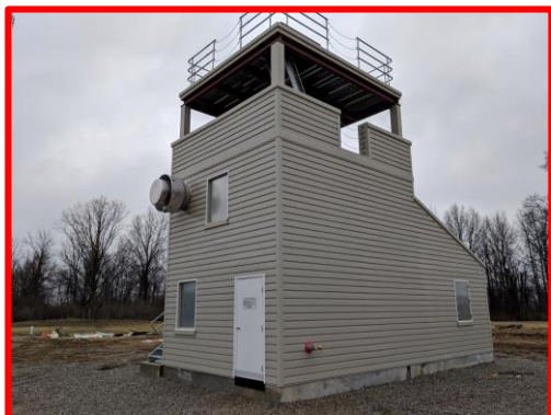
Picture 3: Completed Burn Building
