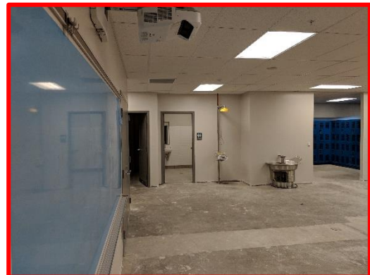
Picture 7: Progress in EMT
