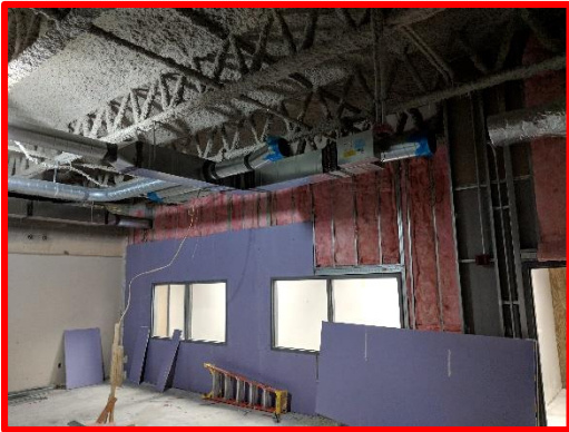
Picture 1: Progress in the New Shared Classroom
