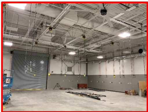
Picture 2: Hung Pendant Receptacles in the Welding Lab
