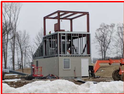
Picture 4: Progress of the Burn Building
