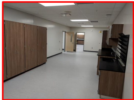
Picture 6: Final Finishes Applied in the Science Prep Room
