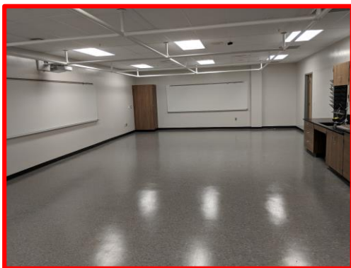
Picture 2: Progress of the General Science Classroom
