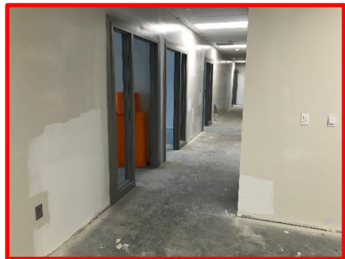
Picture 7: Progress in the East Admin Area Corridor
