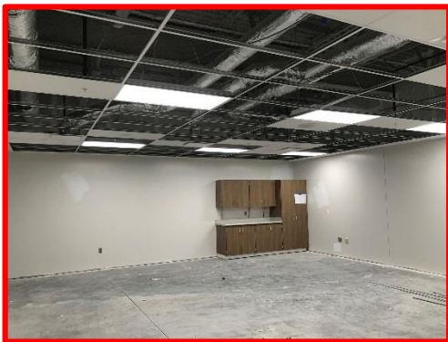
Picture 5: Casework in the East Admin Area Classroom
