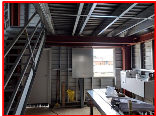
Picture 6: Smoke Machine and Interior Progress of the Burn Building
