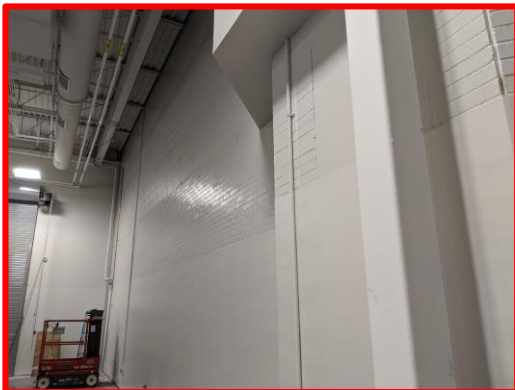
Picture 5: Final Coat of Paint in Fire Service Tech
