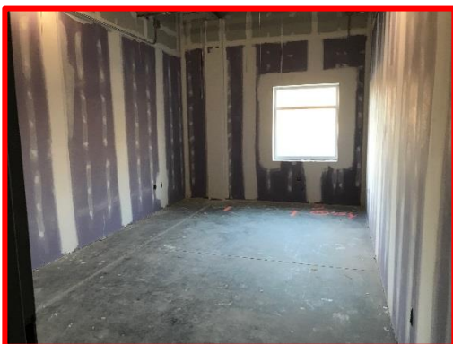
Picture 3: Drywall Finishing in Jack's Future Office
