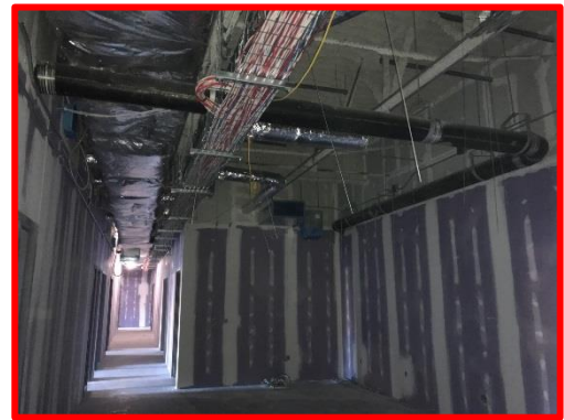
Picture 5: Acoustical Ceiling Wires in the East Admin Area
