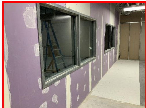
Picture 3: Finishing of Drywall in New Shared Classroom 633
