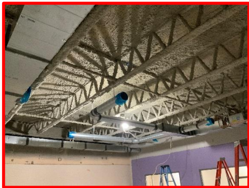
Picture 2: Above-Ceiling Progress in New Shared Classroom 633
