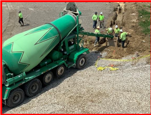
Picture 1: Placement of Concrete Piers at the Fire Storage Building
