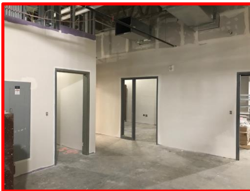
Picture 5: Horn/Strobe in the Fire Service Tech Classroom
