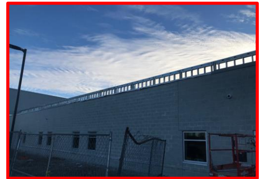
Picture 6: Screen Wall Framing on the East Side of the Building
