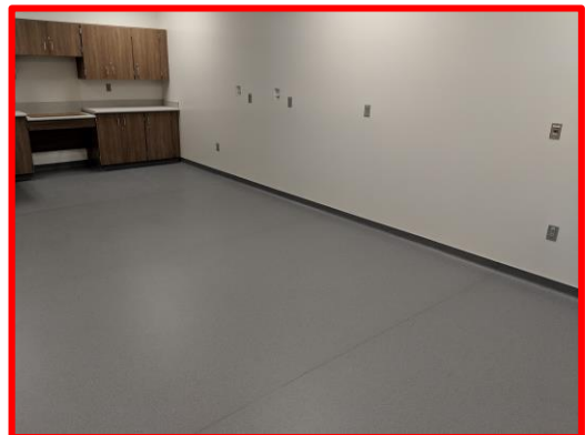
Picture 5: Vinyl Sheet Flooring in The Forum Prep Kitchen
