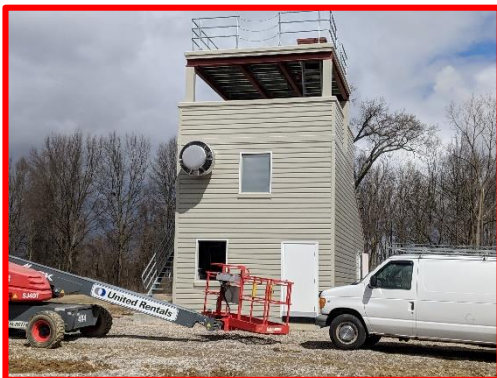
Picture 2: Burn Building Approaching Completion
