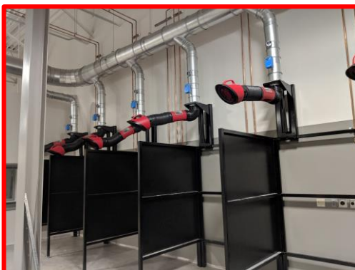
Picture 3: Progress in the Welding Lab
