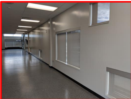
Picture 6: Final Coat of Paint in Fire Service Tech
