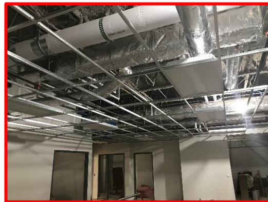
Picture 7: Acoustical Ceiling Grid in the EMT Classroom
