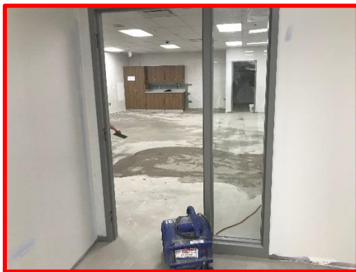
Picture 6: Floor Preparation in Classroom 511
