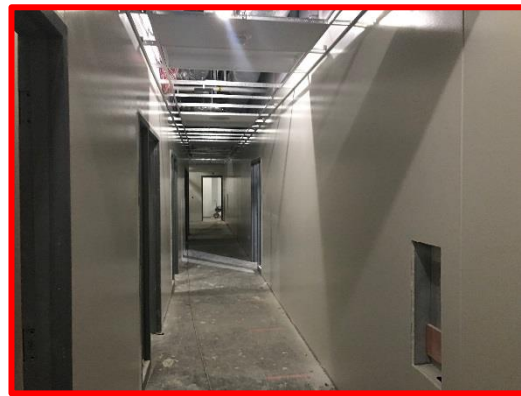
Picture 5: Prime and First Coat of Paint in East Admin Corridor
