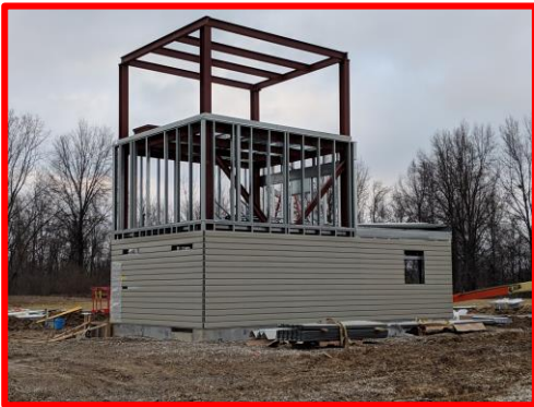
Picture 2: Exterior Metal Panels on the Burn Building
