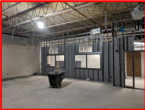
Picture 1: Progress in the New Shared Classroom
