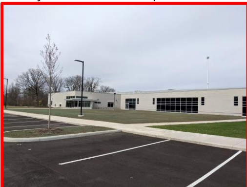
Picture 3: Final Grading at West Entrance
