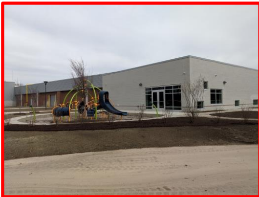
Picture 2: Hydromulching outside of Early Childhood Development
