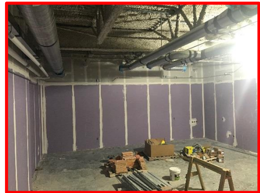
Picture 5: Finishing of Drywall in the East Admin Area Classroom
