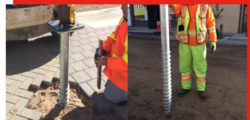
Our ground screw foundations use the natural compression of the earth for strength and stability.
