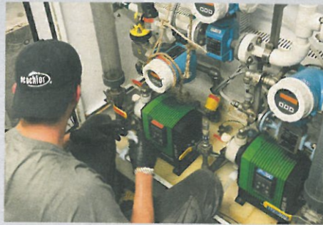
Jonathan Perlich, Chem Resupply Manager on a 'health check' for the chlorine dioxide generator during Chemical Resupply
